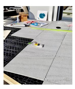
**(Optional)** • If polymeric sand or grouting is to be used, install a geotextile/landscape blanket over SilcaGrates. This helps the sand from falling through during install. If adhesive of tile direct to the Silca Grate is still required, simply cut holes as you go.
