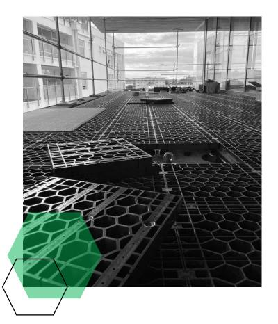
Attach the Silca Grates to joists using X6 countersunk head selfdrilling screws per grate. 10G X 60 410 CSK SQ SELF DRILL WINGTEK.
